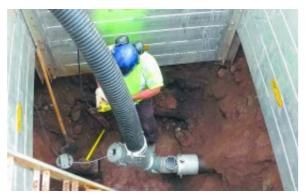
The Tomahawk System, designed by Envirologics Engineering Inc., is a trenchless remediation technology which leaves pipes dry and ready for lining in a few minutes. - Photo: ENVIROLOGICS ENGINEERING INC.
