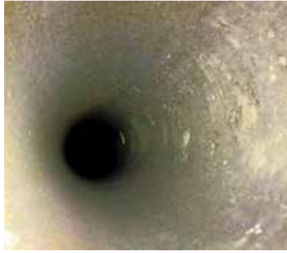
THE PHOTOS ABOVE, FROM LEFT, SHOW THE SAME WATER PIPE BEFORE CLEANING, AFTER A TOMAHAWK CLEANING AND AFTER THE TOMAHAWK BARRIER COATING. THE IMAGES ARE FROM THE JULY 2015 WATERLOO DEMO. CREWS WERE ABLE TO LINE 53 M OF PIPE IN 10 MINUTES.
