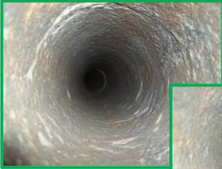
Bitumen liner being removed
