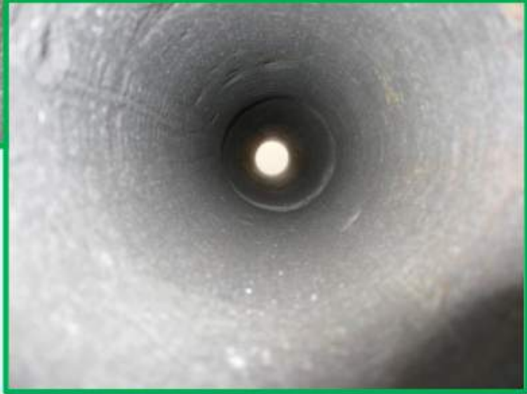
Fully prepared for liner bonding
