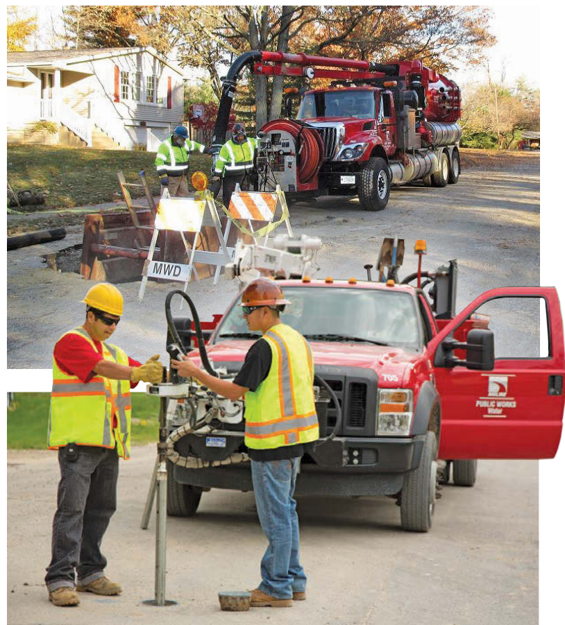
Top Right: A Vactor 7500 pulls the grit from the Tomahawk system through a section of water main. (Photo by Moline Public Works Department) Right: Joe Sammon (left) and Ryan Rangel use a truck-mounted hydraulic valve operator to exercise a valve. (Photo by Mark Hirsch)
