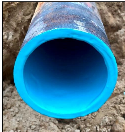
Pictures: Above left, cleaning operations outside of building, above top right, exterior horizontal end of pipe after cleaning, lower right, after lining with Tomahawk BluKote™.
