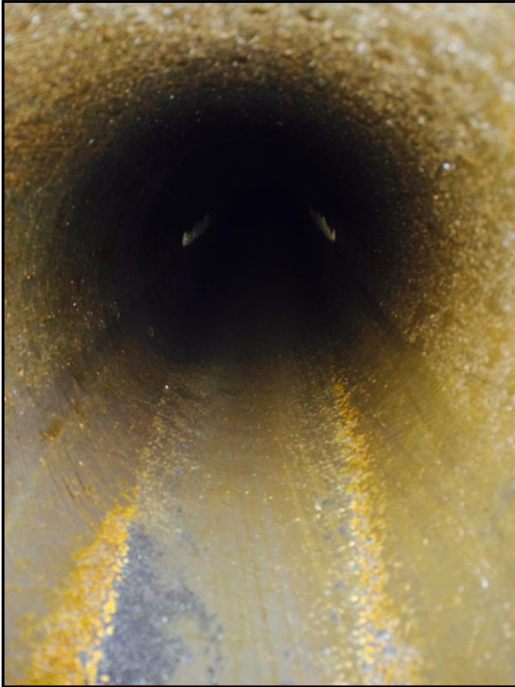
6" CML lined CI pipe, corrosion and bio film removed, dried and lined
