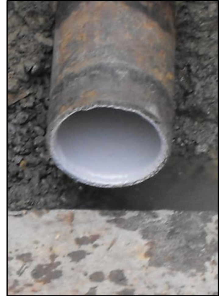
6" CML lined CI pipe, corrosion and bio film removed, dried and lined
