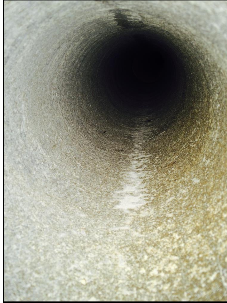
6" CML lined CI pipe, corrosion and bio film removed, dried and lined
